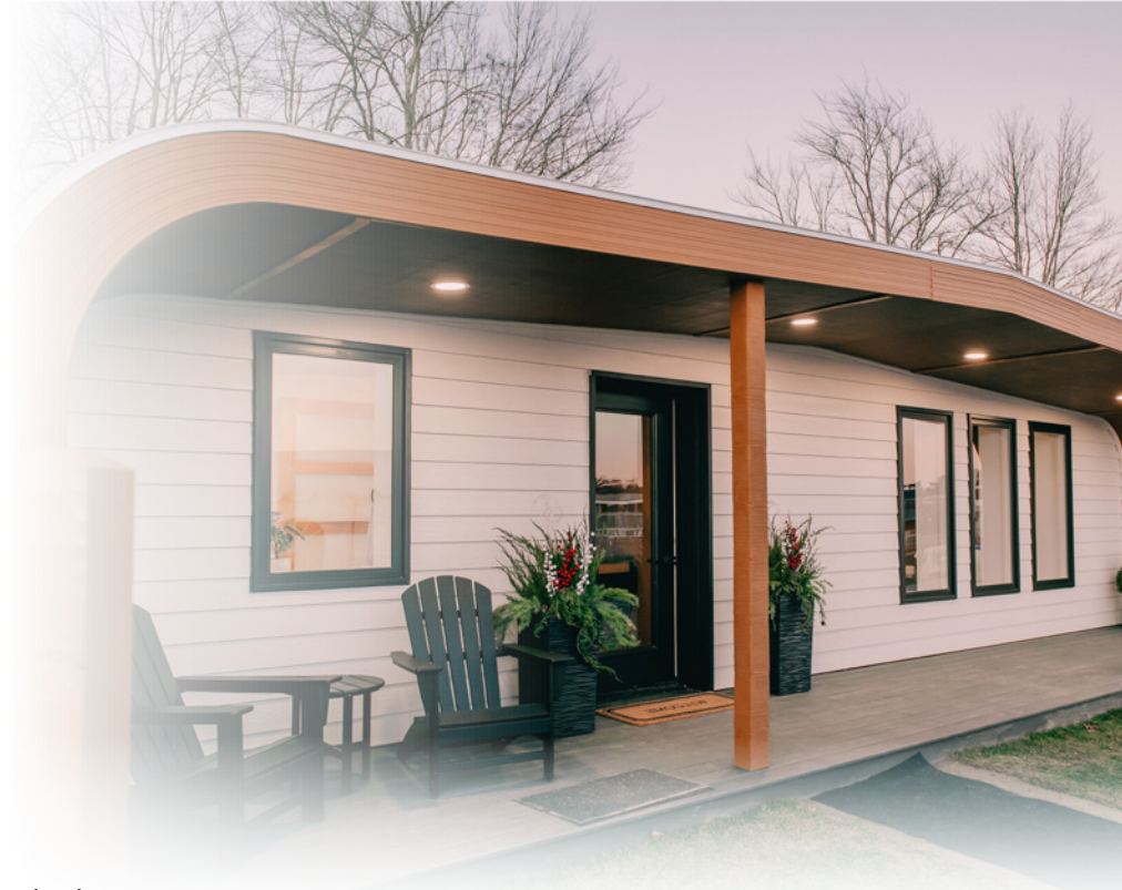
3D-printed bio-based house
